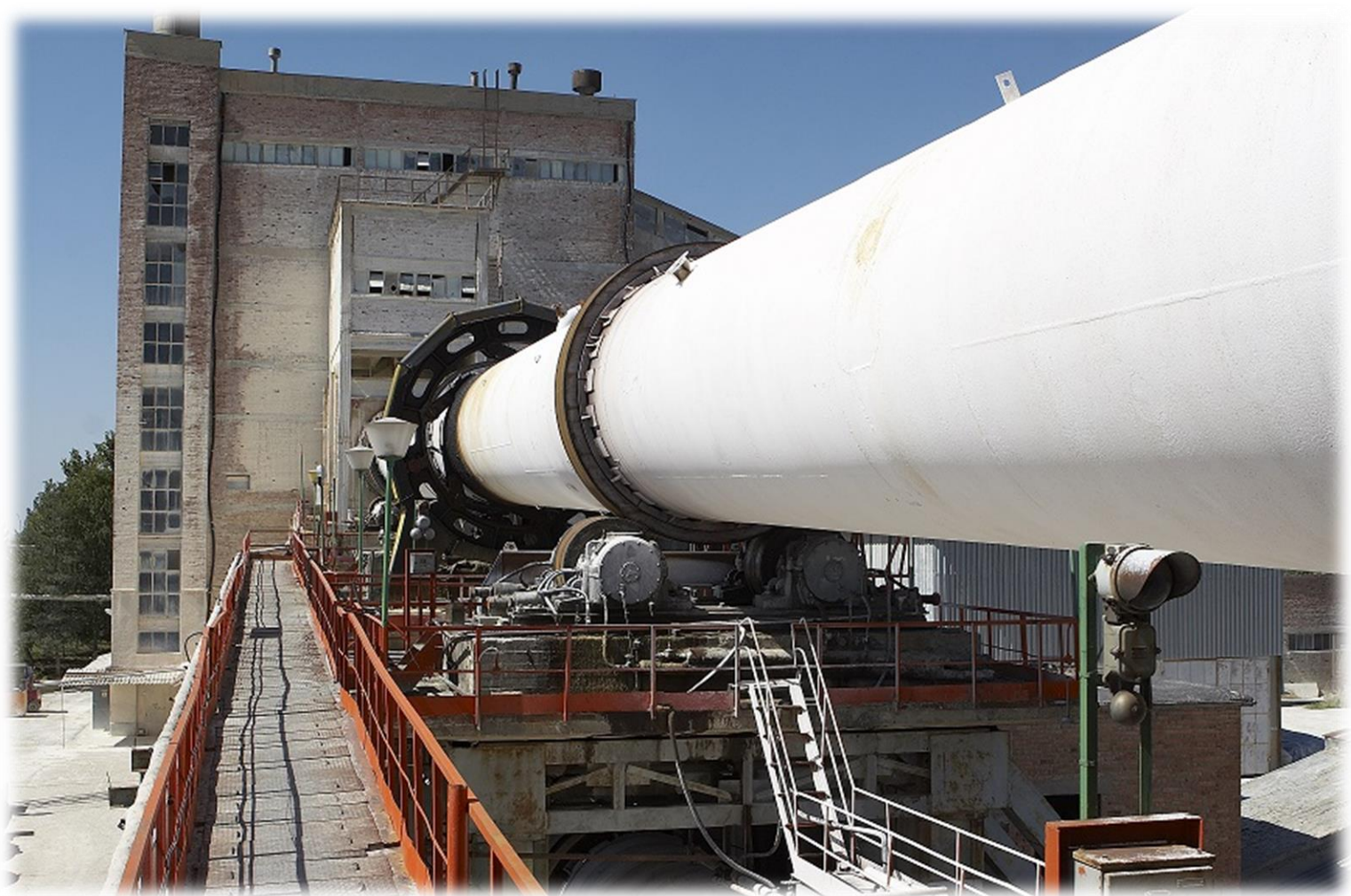
Rotary kiln in Vetovo-Bulgaria, 60 m long
